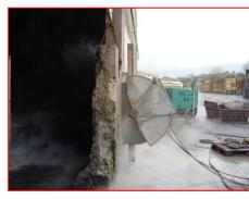
Nash Industrial Services contacted Ram Services and stated that they required a section of reinforced concrete wall 6m high x 2m wide x 375mm thick removing from the Lafarge coal store in their Stoke factory, to allow Lafarge to utilise larger vehicle access.
